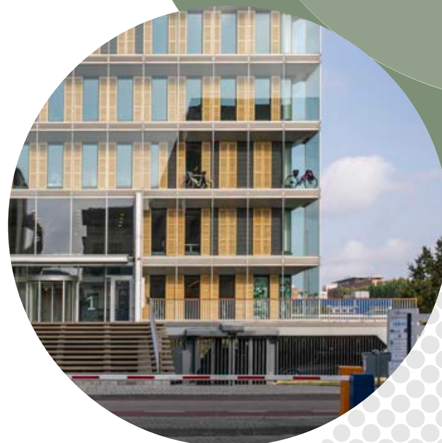
Indoor parking garage
